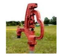
Yard Hydrant – these should have a vacuum breaker or a Reduced Pressure Backflow Device to prevent backflow.
