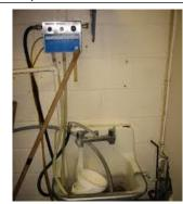
A mop/cleaning sink is present in many homes and businesses. If a vacuum breaker is not installed on the faucet, the non-potable water in the sink could back siphon into the potable water system.
