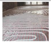
Radiant floor heating – if the system is connected to your home water source, a Double Check Valve Assembly or Reduced Pressure Backflow Device is necessary.
